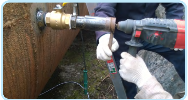
Insertion Transducer Installation
